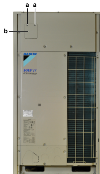
a Screw b Service plate
