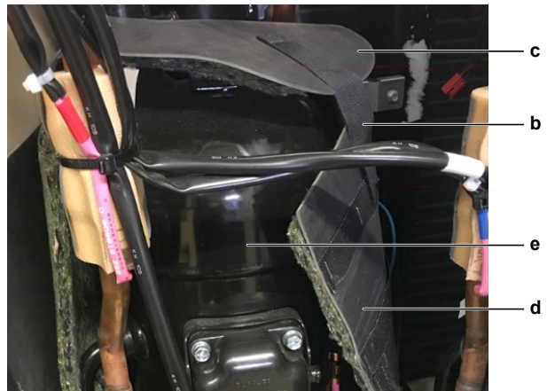
b Strip c Top jacket d Body jacket e Compressor
